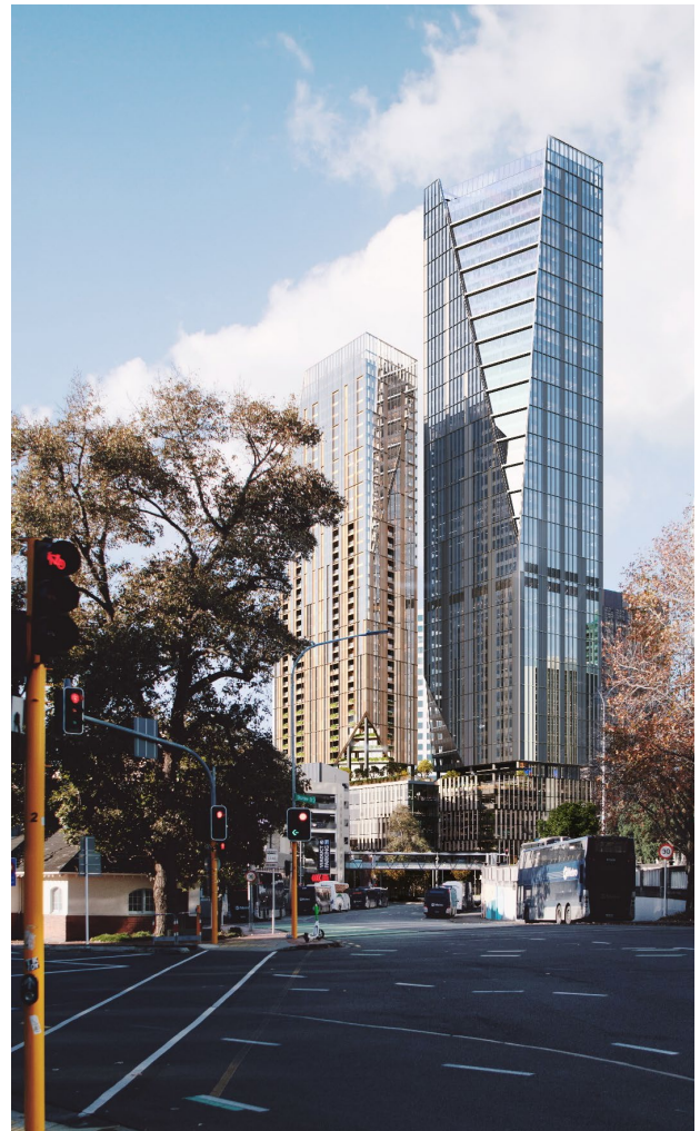
Figure 2.6 Facade detail, texture and colour apparent in this mid-range view along Sturdee Street (Extract from W&M Render 12)
