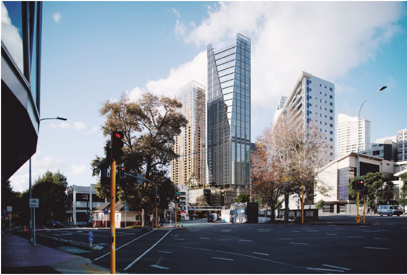
Figure 2.19 Approach view to the city centre along Sturdee Street (Render 12)
