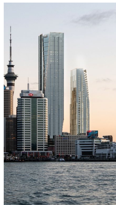
Figure 2.23 View from the north-east on a typical ferry route (Extract from Render 04)
