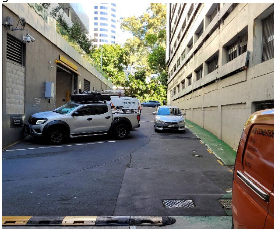
Figure 4.24 View southward towards Federal Street showing. Base and service areas of Aon House on the left, the Downtown Carparking Building on the right.
