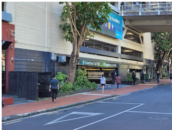
Figure 4.11 Presentation of the existing DTC to Customs Street West, looking east.
