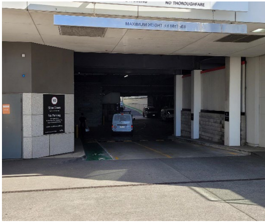
Figure 4.22 View of entry from Quay Street. Relative darkness means this appears uninviting. Pedestrian access is signalled by the painted green line.
