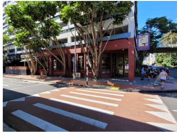
Figure 4.9 South-west corner of the site as it currently presents to Lower Hobson Street, with the corner entry to Monsoon Poon restaurant at right.
